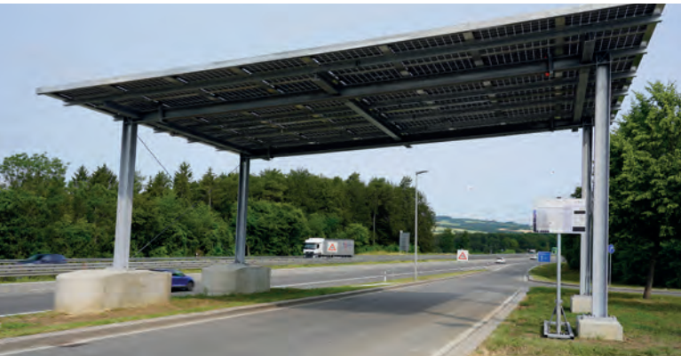
Demonstration of a PV canopy for roads at the Hegau-Ost rest area, Baden-Württemberg, Germany.
