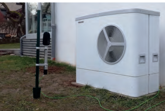
Outdoor air heat pump with additional acoustic measurement technology in front of a single-family house from 1955.
