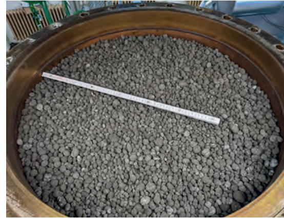
Molten salt / loose filler material storage tank after introduction of filler material.
