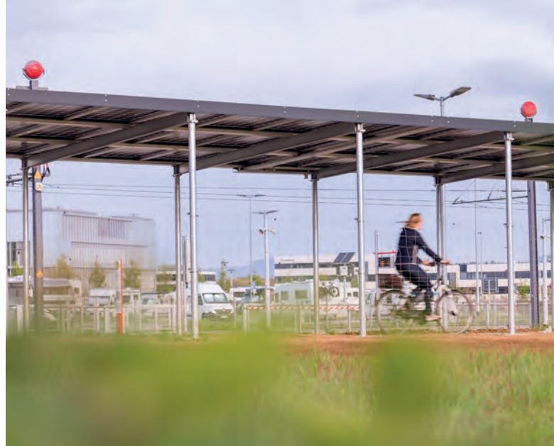
Fraunhofer ISE uses the electricity from Germany's first solar cycleway canopy. The system is located near the Institute and the Messe Freiburg (Freiburg Trade Exhibition site).
